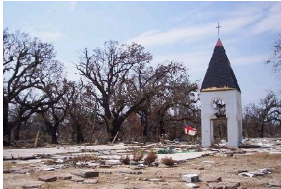
Christ Church after Hurricane Katrina
